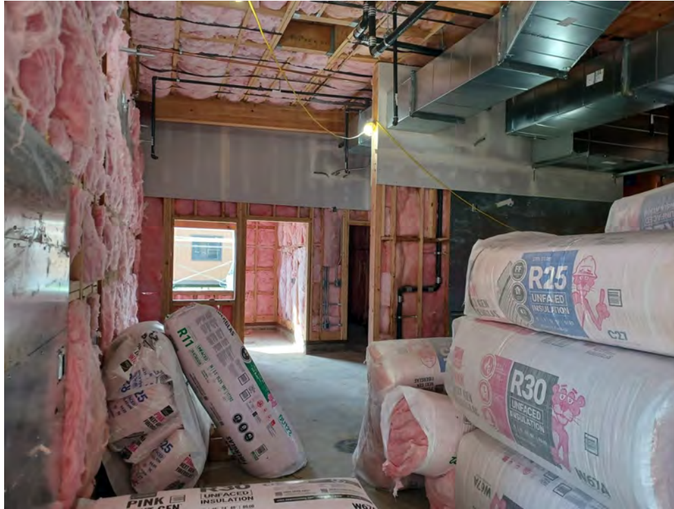
Insulation in progress
