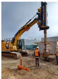
Drilling for Canopy Structure
